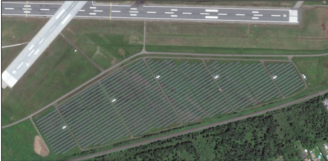
Photovoltaic arrays at Thunder Bay Airport (Google Earth)
