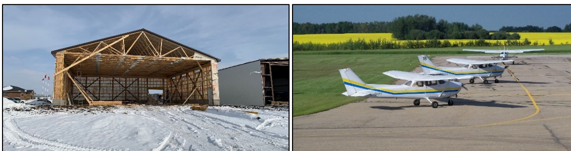
A hangar under construction (left) and flight training aircraft (right)
