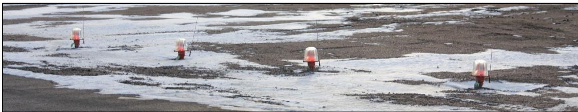
Runway end lights
