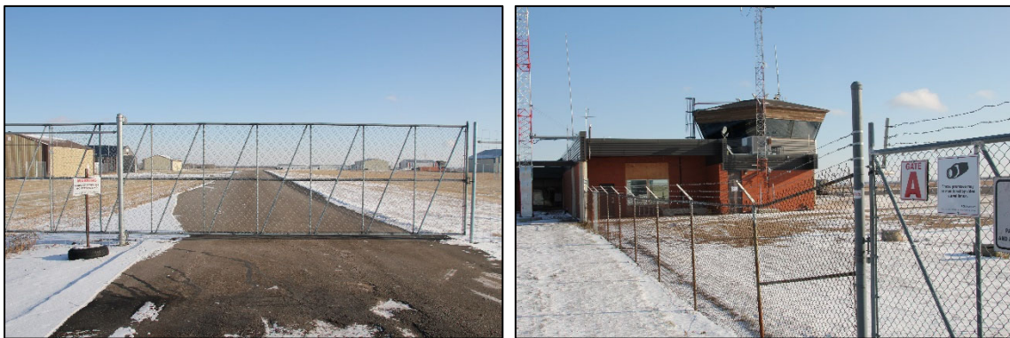
Airfield access gate (left) and perimeter fencing (right)
