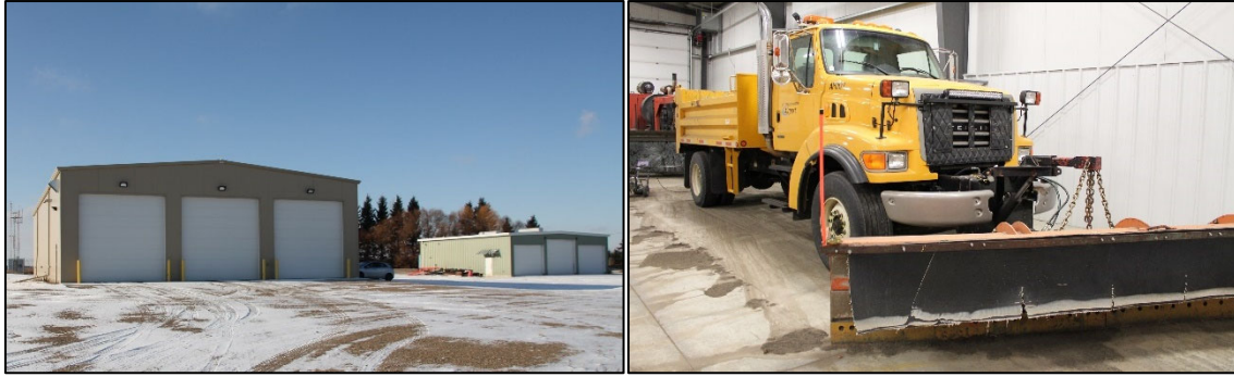
Maintenance garage (left) and a truck with an attached plow (right)
