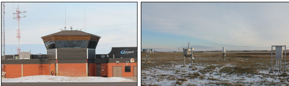
Flight Service Station (left) and Meteorological Observation Site (right)
