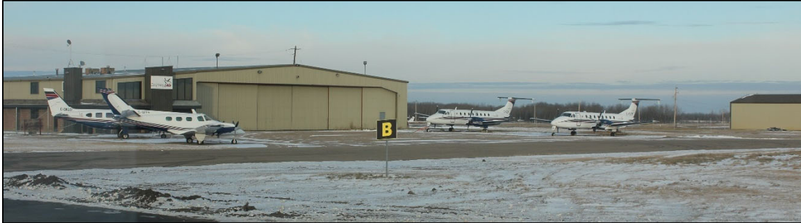
Taxiway B facing northeast
